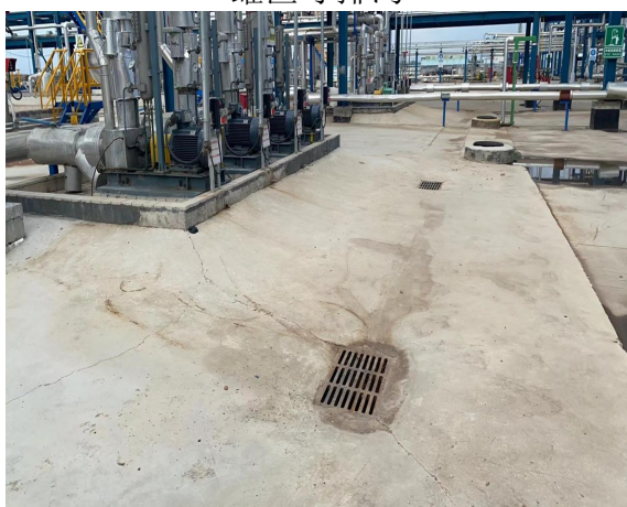
装卸区导排沟围堰
